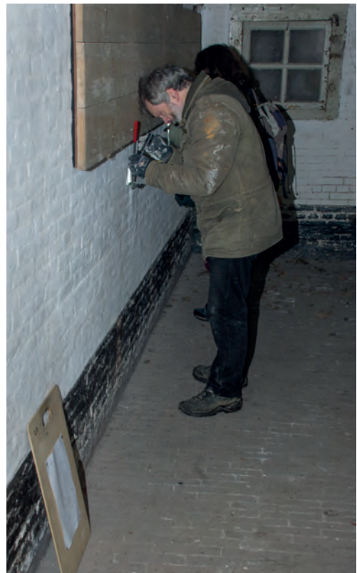
Figure 3. Inspection of Fort Honswijk (20).
