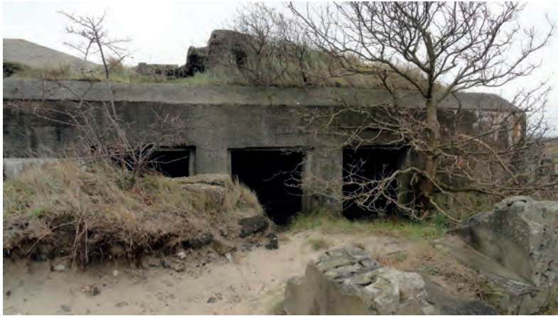
A bunker on Kop van Schouwen (prov. of Zeeland, the Netherlands) that was previously buried under sand. Photo: Kees Mostert.
