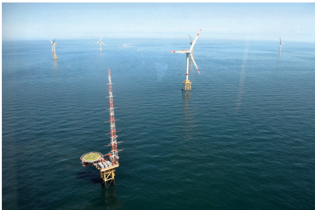
Figure 2. The research platform FINO 1. Photo: Reinhold Hill.
