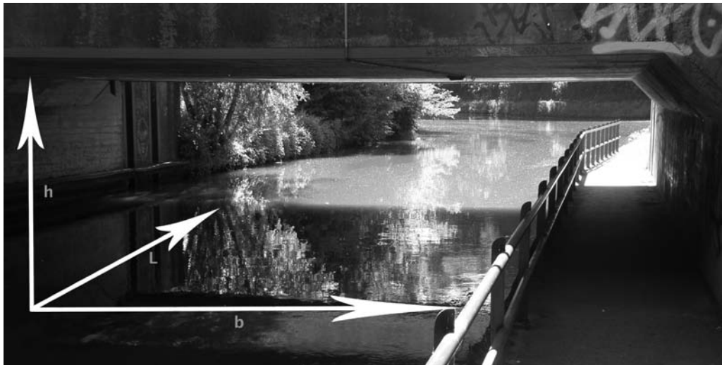
Photo 4. Length (L), height (h) and width (b) of a culvert. Photograph: M. Boonman
