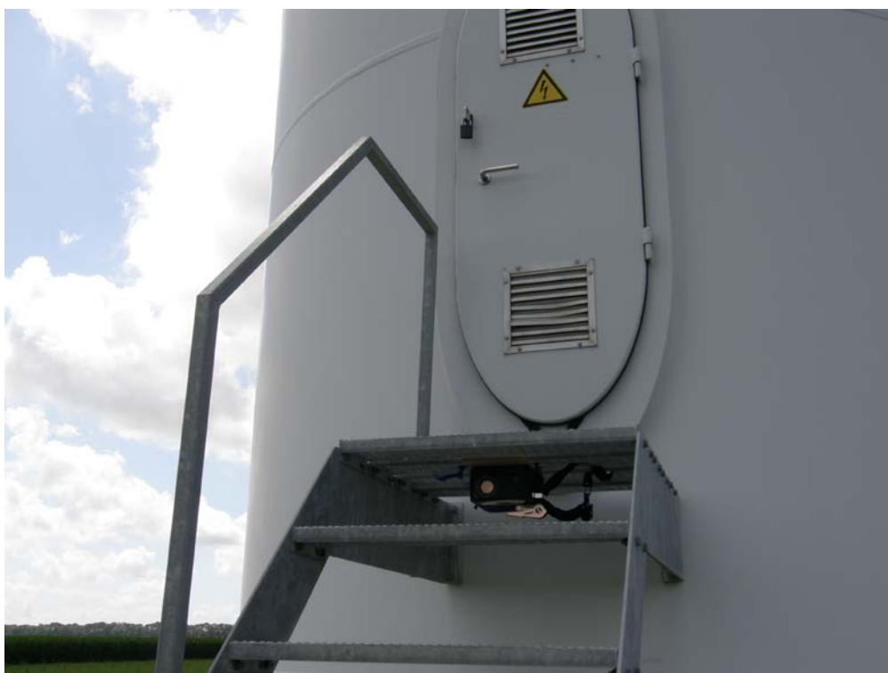
Figure 4.4 The bat detector situated at ground level.
